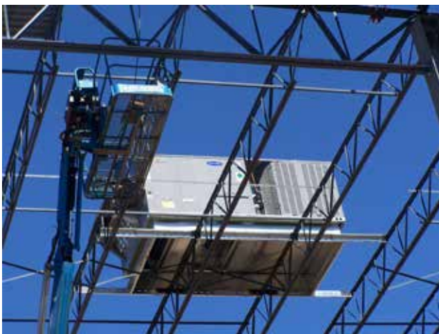
▲ A QuickFrame roof penetration before deck installation...
